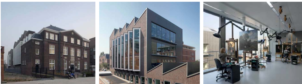
Image 1: The Atelier Building, Hobbemastraat 22 in Amsterdam, will house the core of the knowledge center Science for Arts of the Netherlands . Currently on this site there is already collaboration taking place between the Cultural Heritage Agency, the Rijksmuseum and the Conservation and Restoration training program of the University of Amsterdam.
