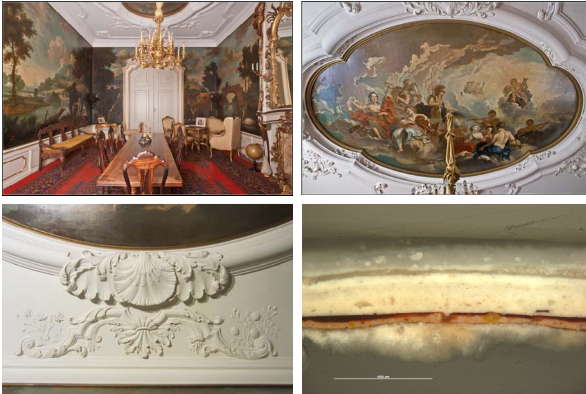
Image 7: Recent NWO-funded research shows that plaster ceilings originally often had a colorful finish in imitation of unusual types of wood and stone. Nowadays these original finishes are almost always hidden from sight by a series of later paint layers. The current bright white plastered ceiling in the salon from Huize de Dieu (1744) in Alkmaar originally had a brown-red finish, which presumably imitated mahogany. The cross-section shows a pink paint layer covering the plaster, with a transparent brown-red layer above it (both part of the original finish). On top of this is a thick series of later white overpaint layers (research: I. Verslype, H. Sigmond; TUDelft, RCE, Rijksmuseum, NWO).
